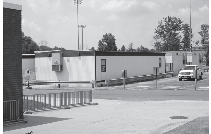
Modular classrooms (trailers) currently house eight classrooms at the edge of the parking lot, outside the main OFHS building.
